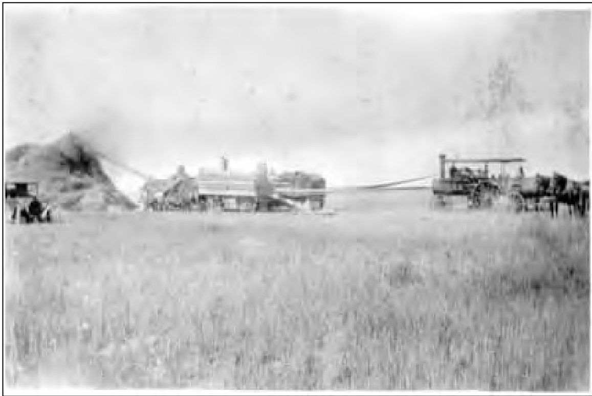
Wheat threshing circa 1910. Bernhard Harder and his brother John owned the machine pictured in these photos. Bundles of harvested wheat were fed into the belt driven thresher that separated the grain from the straw which is being blown into the stack on the left of the upper photo. In the lower photo note the netting on the horses to keep flies at bay. Photos: From the collection of John B. Harder.
