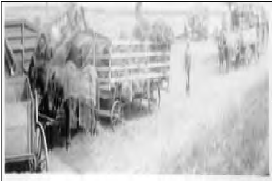
Wheat threshing circa 1910. Bernhard Harder and his brother John owned the machine pictured in these photos. Bundles of harvested wheat were fed into the belt driven thresher that separated the grain from the straw which is being blown into the stack on the left of the upper photo. In the lower photo note the netting on the horses to keep flies at bay. Photos: From the collection of John B. Harder.
