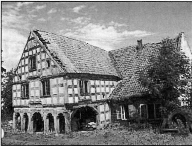
A house in Heubuden built in 1798 for Johann Epp. Source: Catalogue of Monuments of Dutch Colonization,
