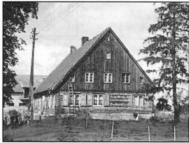
A house in Heubuden built in the early 19 th century. Source: Catalogue of Monuments of Dutch Colonization.
